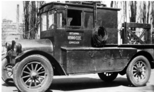
Hydro Electric Car - 1945
